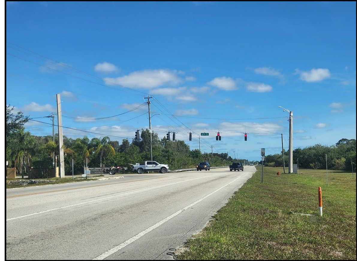
Intersection of CR 510/85 th Street and 87 th Street (Pre-Construction)
