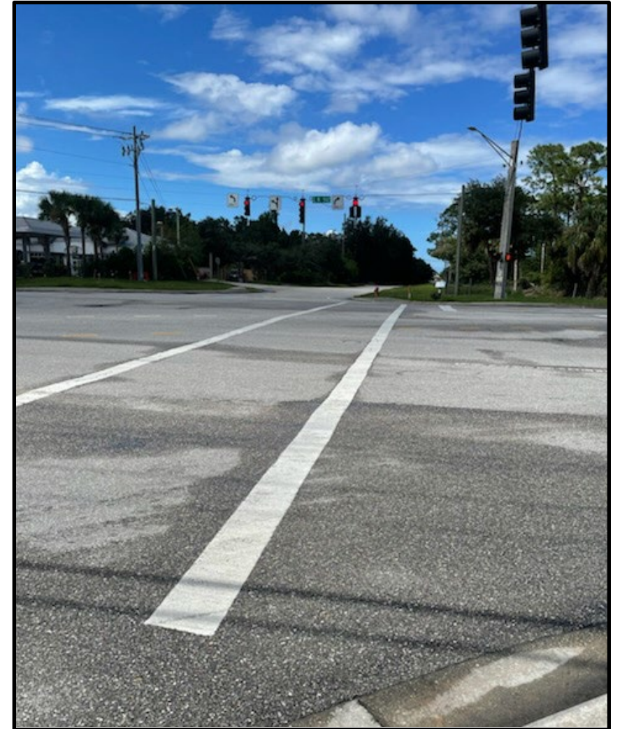
Intersection of CR 510/85 th Street and Hammerhead Way (Pre-Construction)
