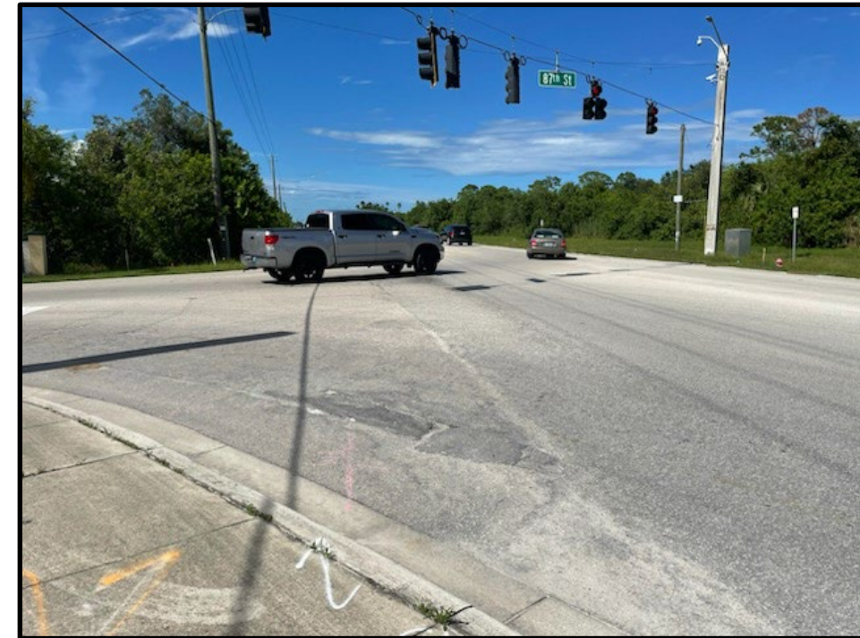
Intersection of CR 510/85 th Street and 87 th Street looking north (Pre-Construction)
